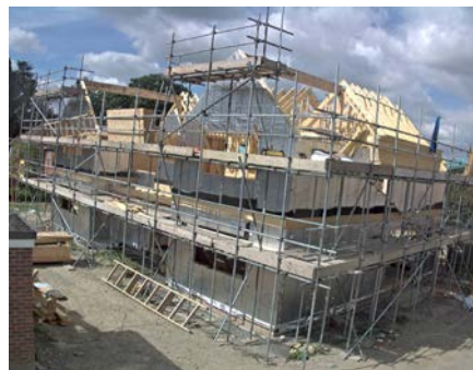
Within days, the wall panels and roof trusses are in place.
