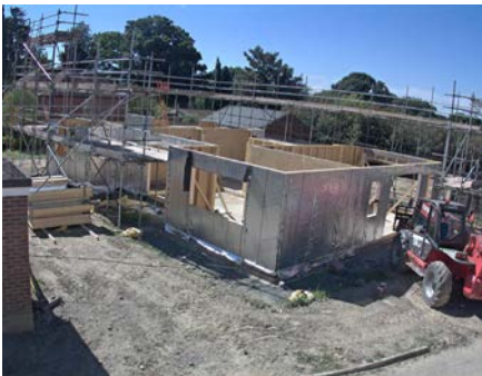
The ground floor external wall panels are quickly erected.
