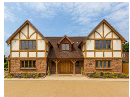
After completion of the internal works you have achieved your dream home.
