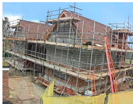
Followed by the external cladding.
