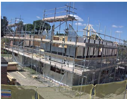
The first floor external wall panels follow shortly.
